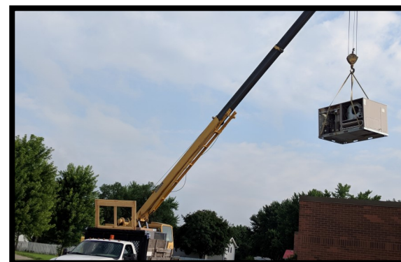
Final stage of placing new AC on roof.
